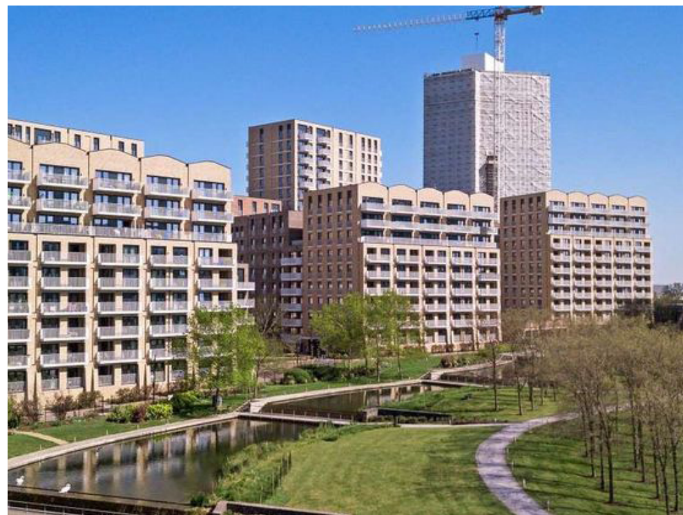
Figure 7: Regency Heights, Lakeside Drive
