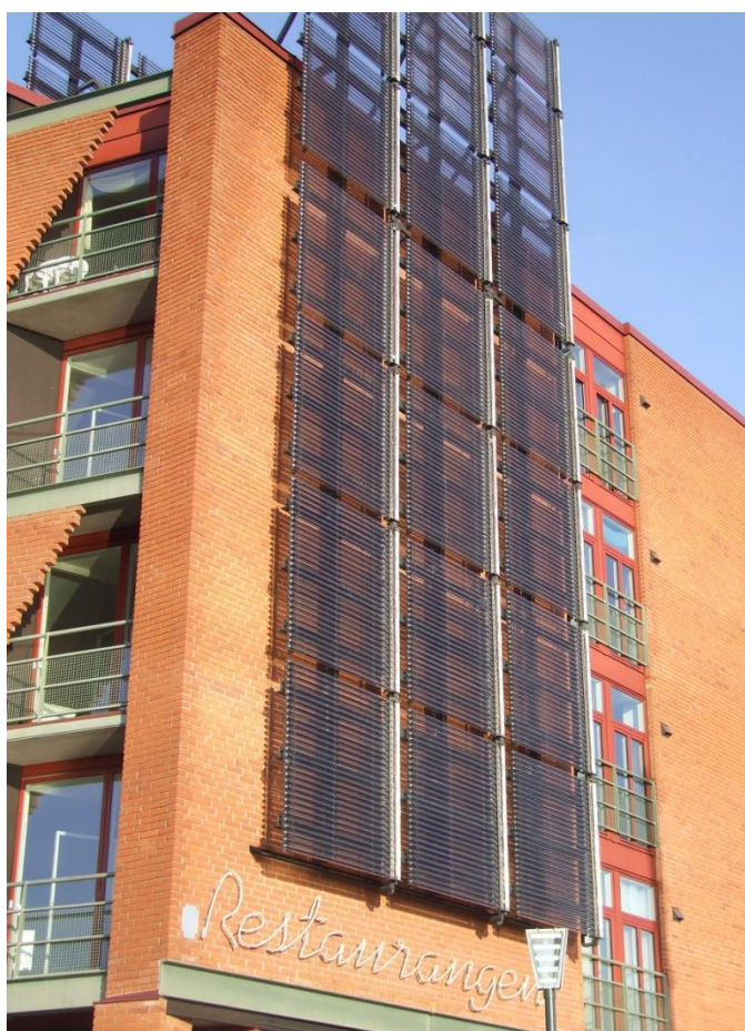
Figure A.2.3. Evacuated Tube Solar Thermal Collectors on Unshaded Facade (Western Harbour, Malmö, Sweden)
