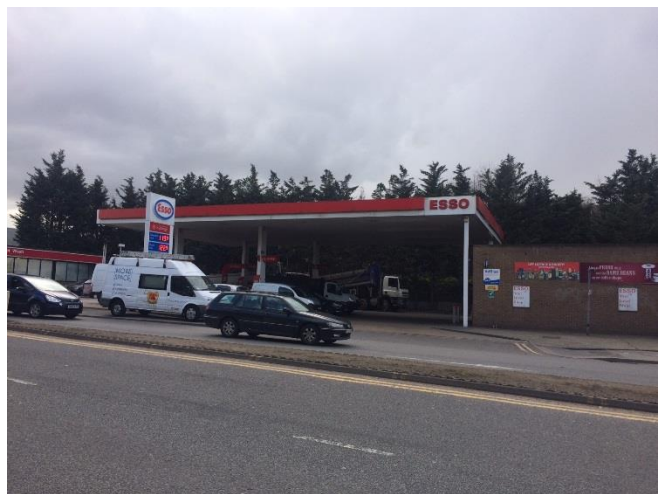
Esso garage to the east of the site
