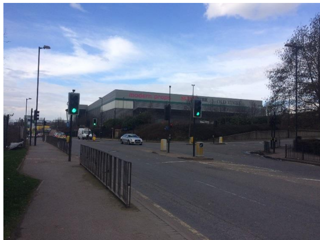
View north along Abbey Road
