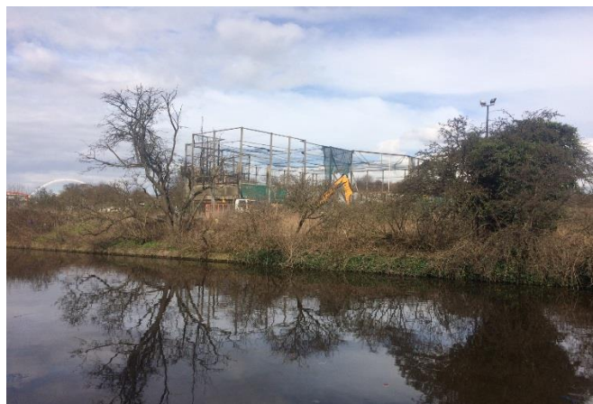
View across the canal (west elevation)
