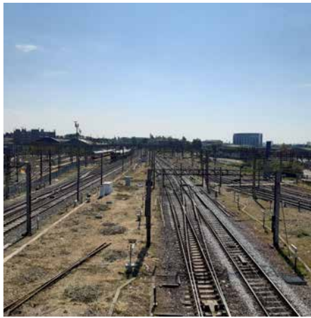
Vantage points from transport bridges – (Old Oak Lane, near Willesden Junction station)
