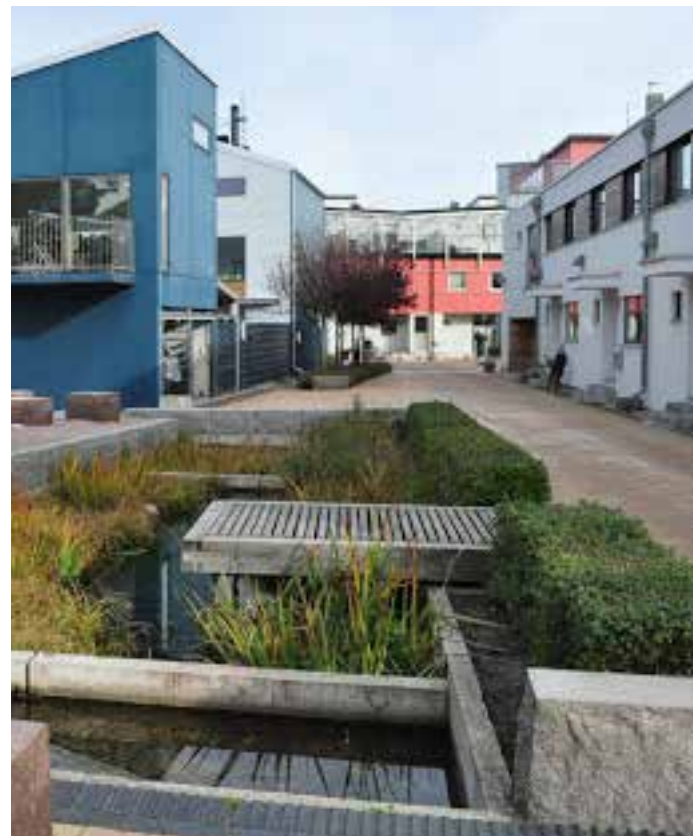
SUDs integrated into residential streets, with planting, seating and viewing platforms in Augustenborg, Malmö (Sweden)
