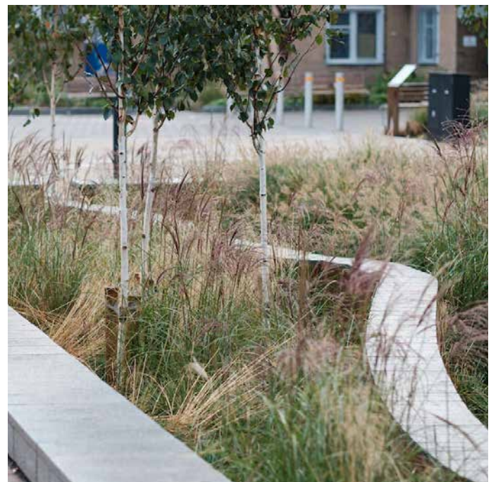
SUDs planter in an urban setting, using robust but permeable edges in White City, West London
