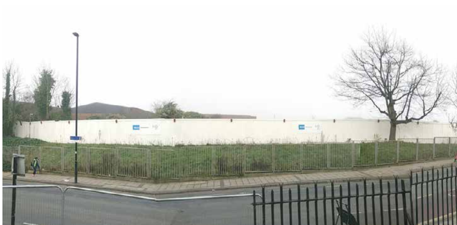
Significant borders with adjacent development sites (HS2 land on Victoria Road)
