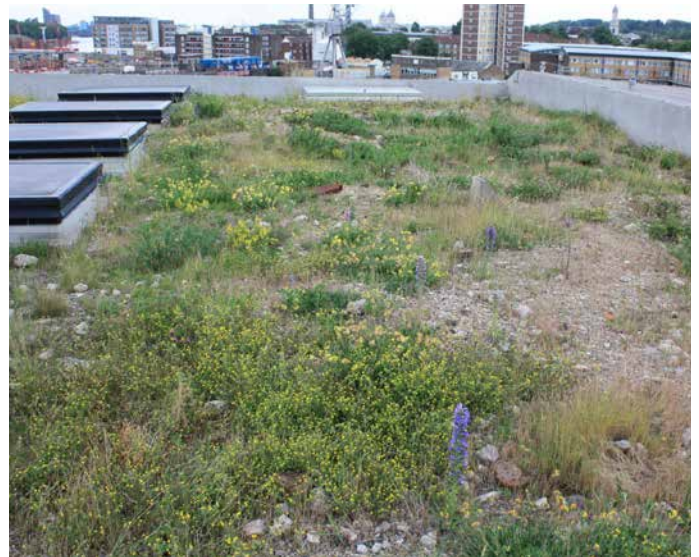
Biodiverse roof of the Laban Centre, Deptford, using rubble waste and locally collected seeds
