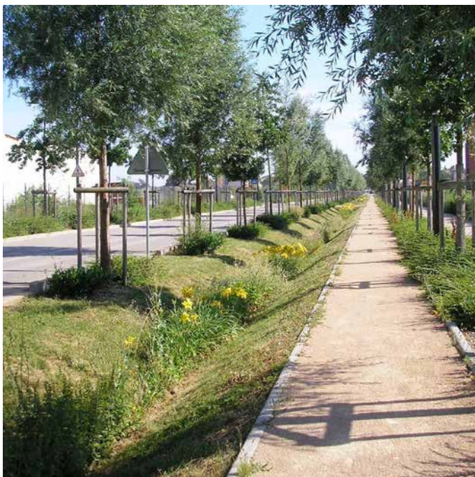
A linear swale running the length of a commuter cycleway in Sathonay, near Lyon
